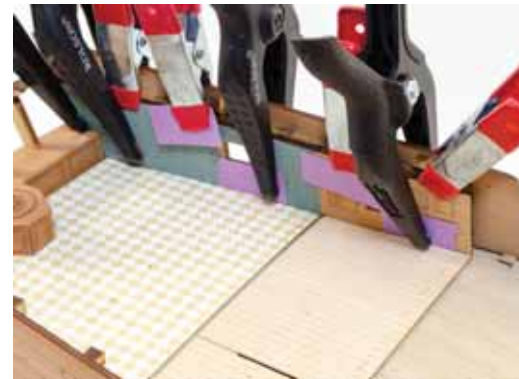
425. The sidewalls can now be glued into place. Use paper etc. to make sure the clamps don't mark the paint and varnish.
