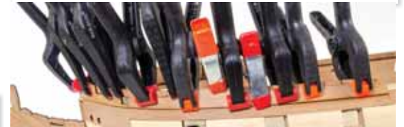
206. Carefully align and glue each part to the upper outside bulwarks at the bow. These will need to be clamped well to ensure full contact. NOTE: You may wish to soak these in water for 30 mins and temporarily clamp into position first. If you do this, then you MUST leave the parts to dry for 24hrs first before gluing them as they will have expanded during soak.
